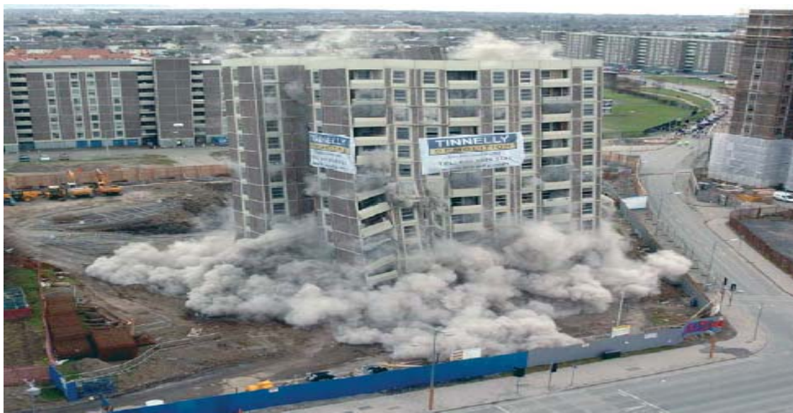
Demolition underway in Ballymun. Photo: www.brl.ie
